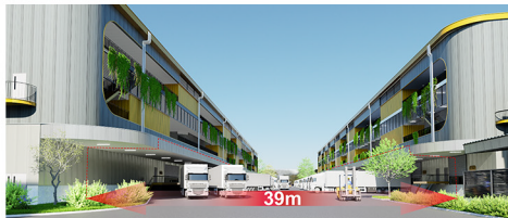
39m-wide internal road
